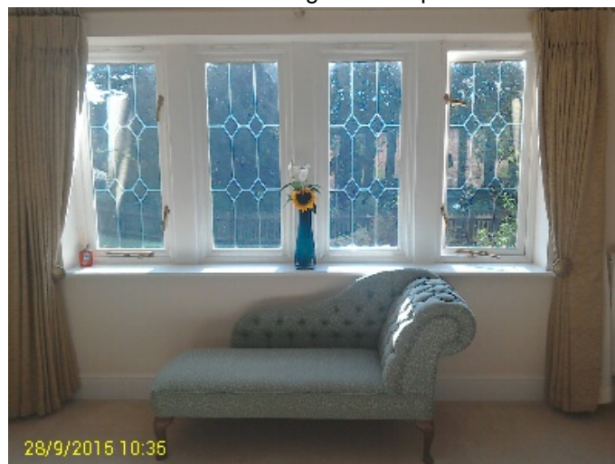
Windows-Wooden Framed glass lead panels
