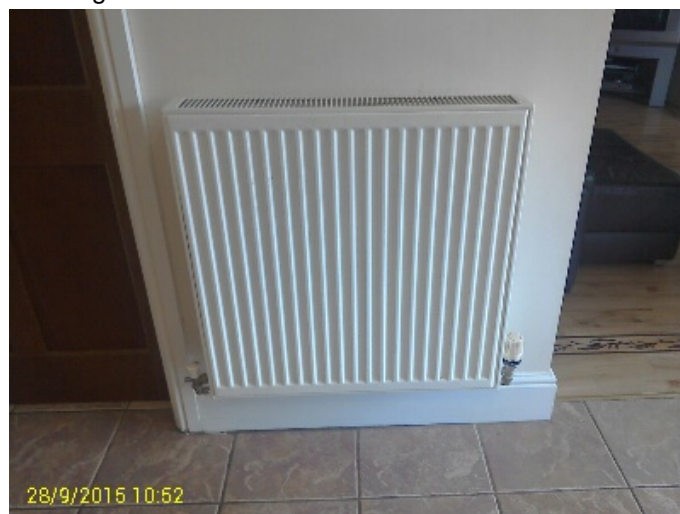
Heating-Wall Mounted Radiator
